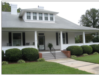
Olive-Seymour-Mills House Billy and Susan Mills 107 South Salem Street
